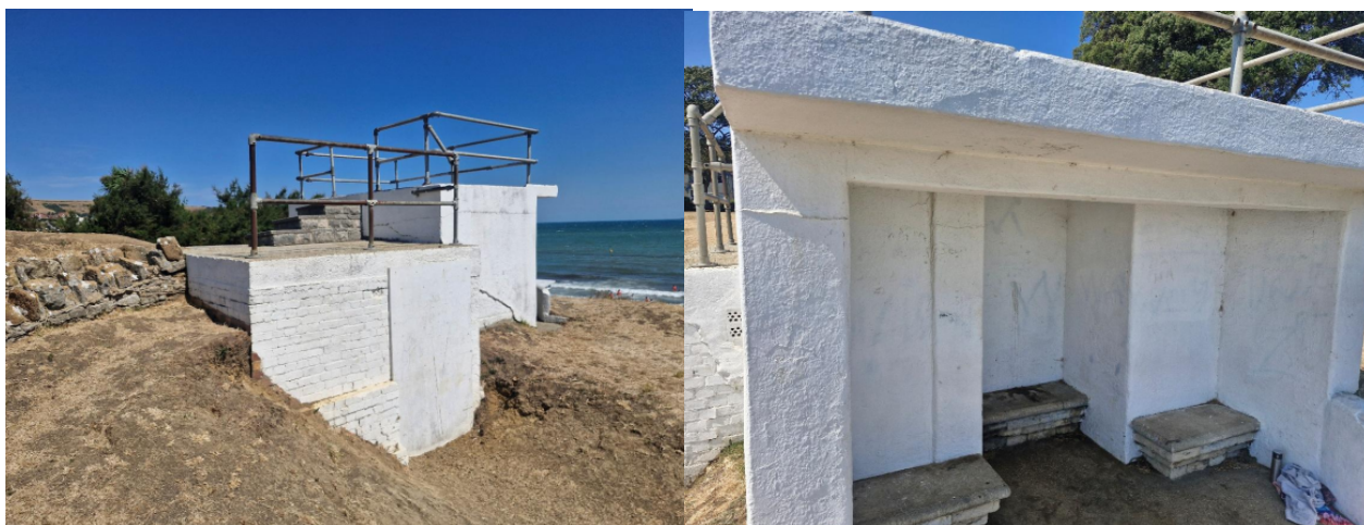
Figure 1 - Images of the existing gun emplacement, taken before it was fenced off for safety reasons.
